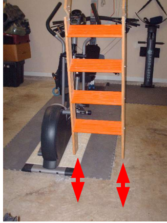
Folding attic stairs to short for the ceiling height.
